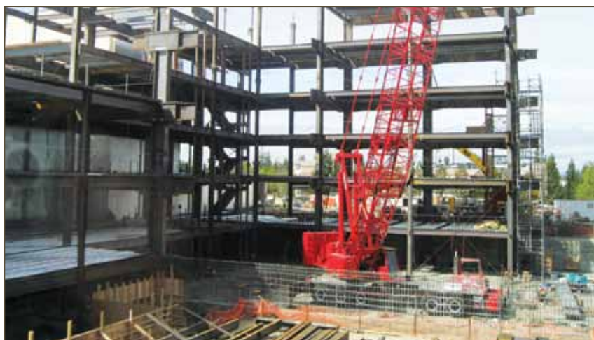
Steel began rising on March 17, 2008 and ended with the topping out ceremony on April 11, 2008. Each of the horizontal beams is 29 feet long and weighs 1,015 pounds.
