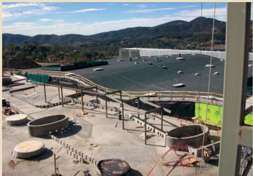
One-way truss system (left) and rolling green roof construction (right) at Palomar Medical Center West
