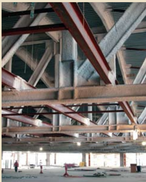
One-way truss system (left) and rolling green roof construction (right) at Palomar Medical Center West
