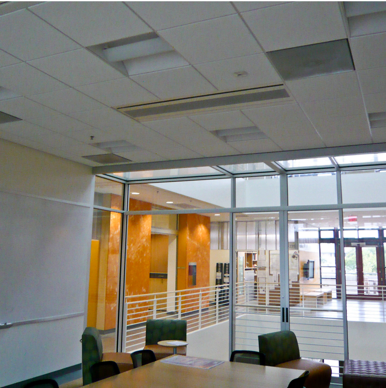
Active Chilled Beam HVAC in Conference Room , Y2E2 Building, Stanford University
