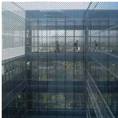
San Jose Joint Library: Fritted glass with a silkscreened pattern reduces glare in south windows while keeping vistas open.
