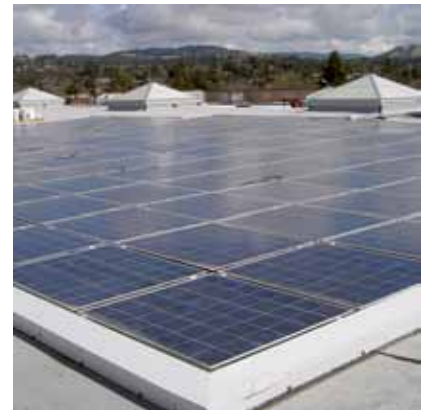
Doyle Library: photovoltaic panels feed power back into the campus grid reducing utility costs.
