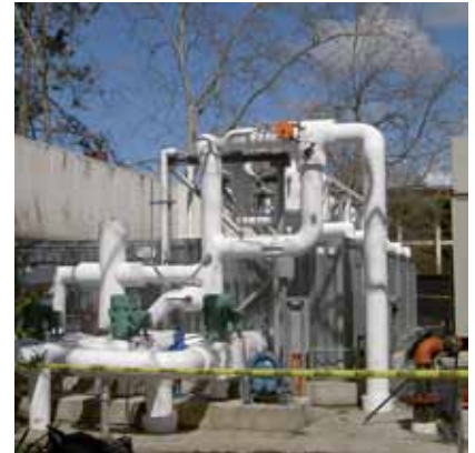
Doyle Library: thermal energy storage units make ice for cooling during off-peak evening hours.
