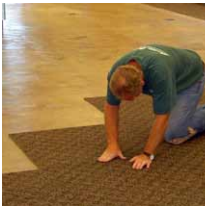
Doyle Library: carpet tiles can be replaced at high wear areas.
