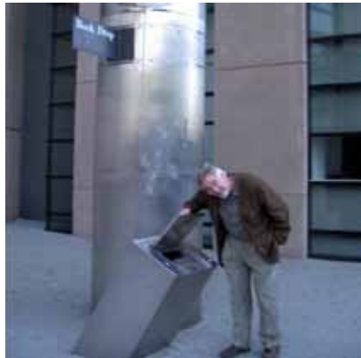
Vancouver B.C. Public Library: an exterior book drop delivers materials to the basement level of the library.
