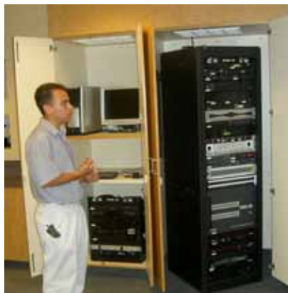
Riverside CC: A video conferencing suite has it's own closets for switching and playback equipment. Note AC vents at tops of closets.
