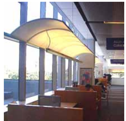
San Jose Joint: Sail like canopies help reduce glare at exterior work stations. They are also reflectors for electric lighting fixtures.
