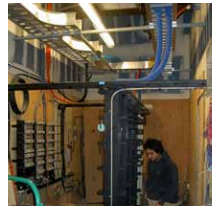
Doyle Library SRJC: large signal closets are the hub for telephone and computer wiring and the fiber optic backbone.
