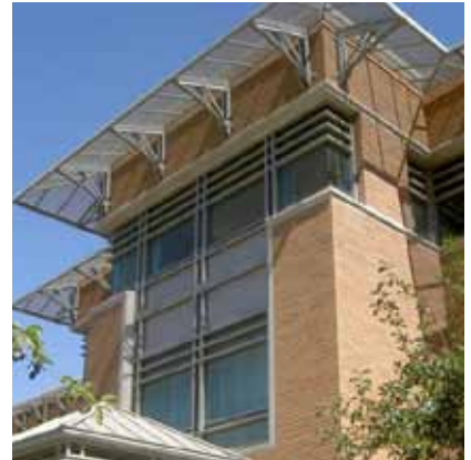
U.C. Riverside Science Library: South facade at entry. Horizontal shading devices help give articulation to the facade.
