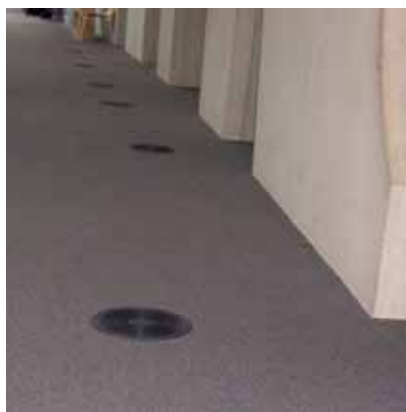
Salt Lake: floor outlets are part of a displacement ventilation system.
