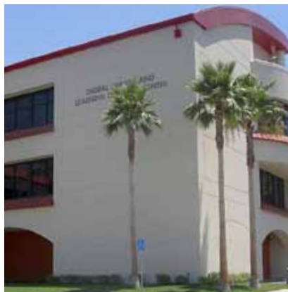
Riverside Community College: stucco is a cost effective and durable material, but it needs periodic painting.
